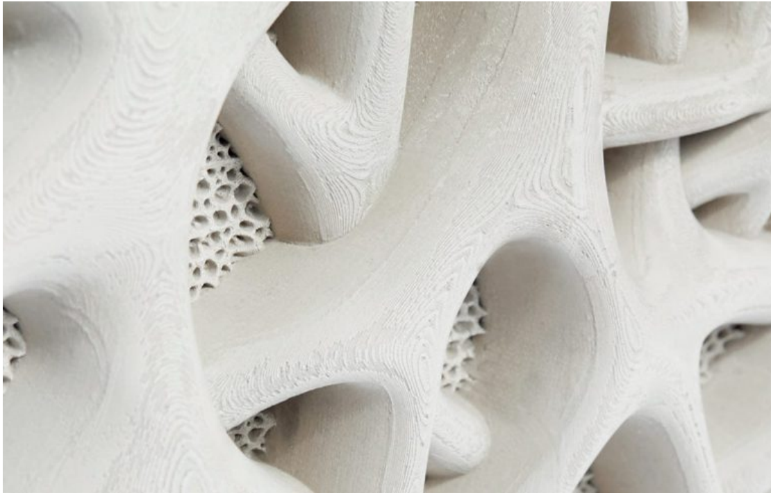
A close up of the sea wall structure, which is designed to encourage habitation by marine life. (Image: Volvo)
